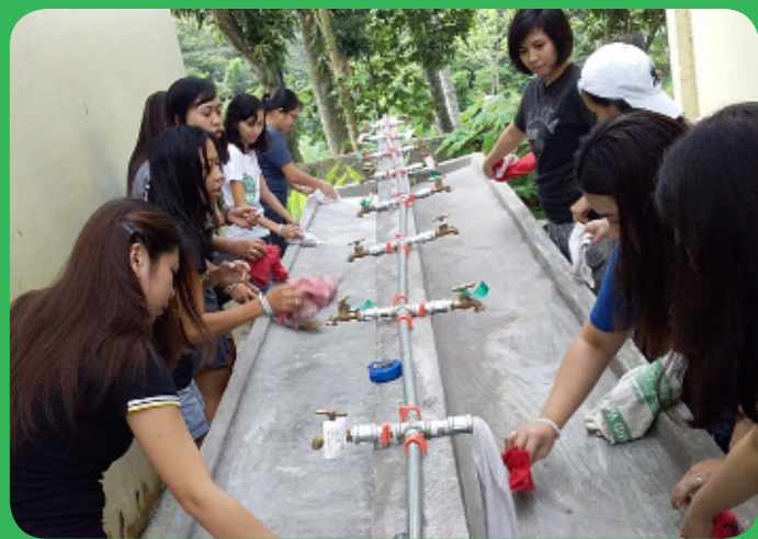
Construction of washing facilities for public school students.
