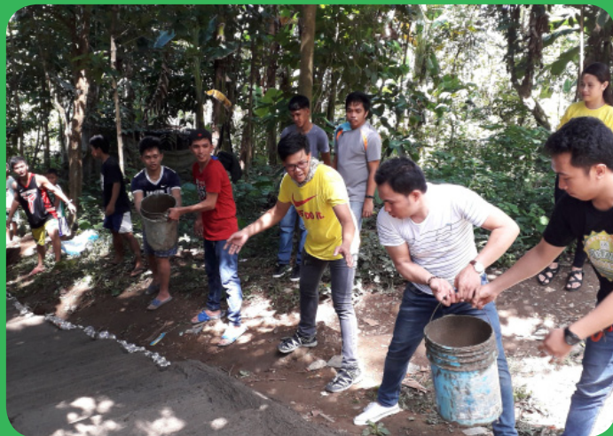
Building of proper walkway for students who live near Taal Lake.
